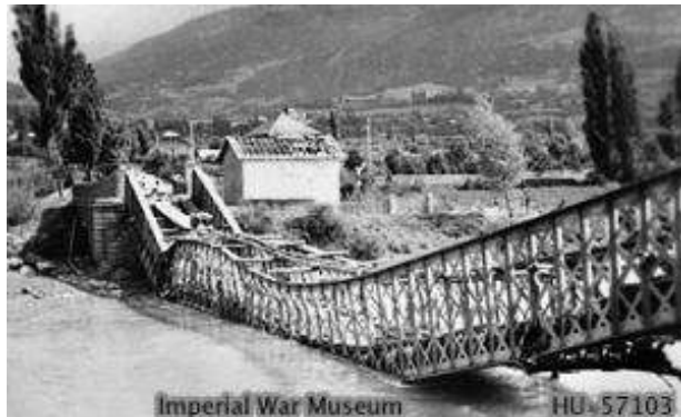
Bridge in Haute-Savoie, France, destroyed by French resistance fighters. Photo courtesy of the Imperial War Museum.
